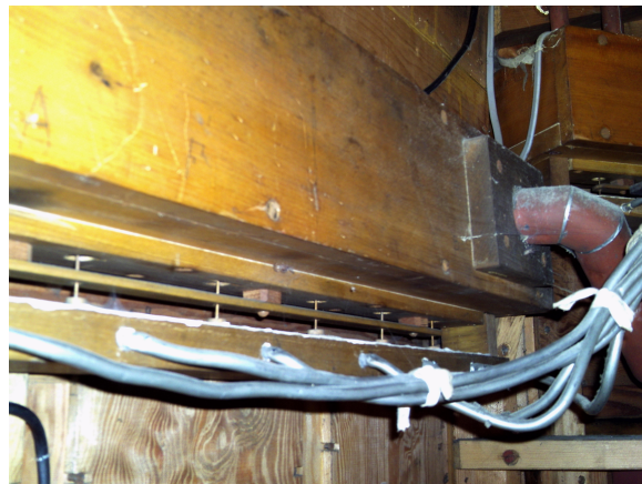
Fig.2 - The same lead tubes under the offset chests under the façade pipes.
